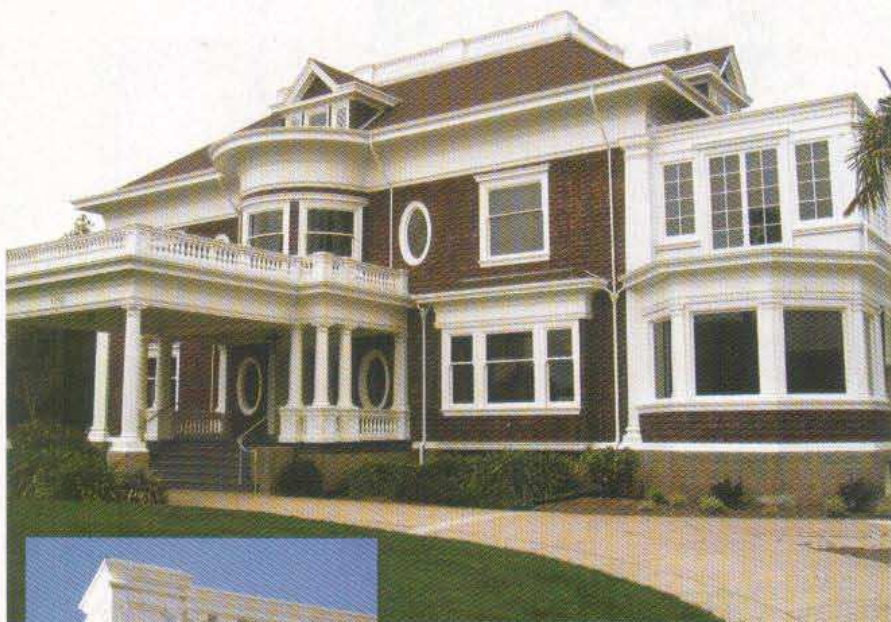
PHOTOGRAPHS COURTESY OF ANDREWS AND THORNEY CONSTRUCTION
