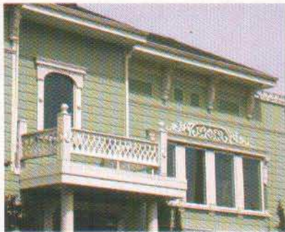
This home on Portrero Hill in San Francisco originally had flat siding and little else. Eric designed the scrollwork, dentil moldings and balcony balustrade.
