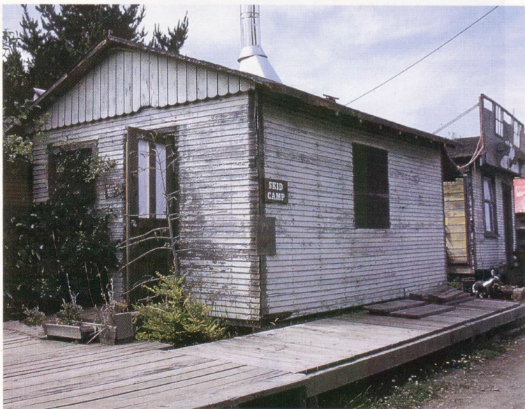
This "skid row" house served as a bunkhouse. Note the platform which is "skidded" with houses aboard.
